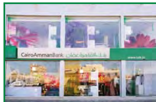
Zarqa Branch - Army Street
